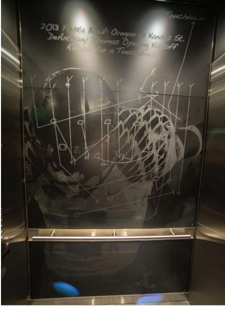
Moon Shadow Glass provided an array of custom-designed interior glass products, including photo-etched panels used in the building's elevators. The company also fabricated four six-panel mirrors with a different scene on each floor.
